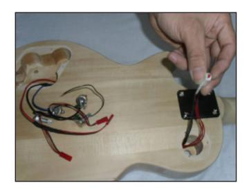
Then put the potentiometers on the right positions as shown in the following picture. The Tone and Volume potentiometers on the downside should be connected to the neck pickup. The Tone and Volume potentiometer on the upper side should be connected to the bridge pickup.
